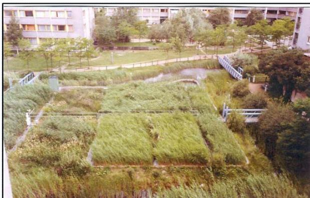
**Figure 5. Constructed wetlands used to treat greywater from a housing development in Berlin, Germany.**
